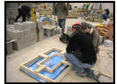
Laying out the foundation
